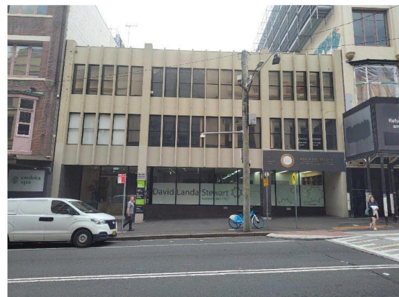
Picture 2 View of the façade along Bay Street
